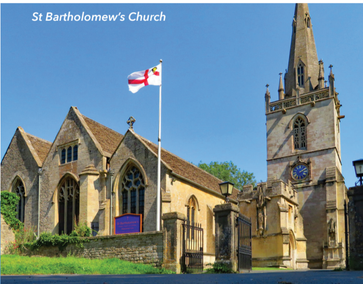
St Bartholomew's Church
