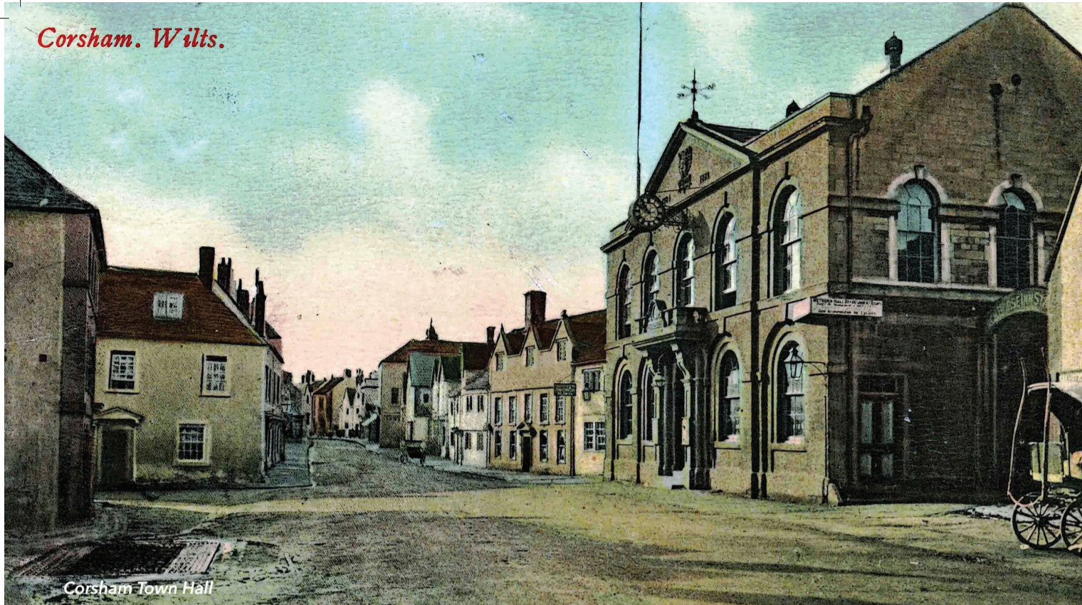
Corsham Town Hall
